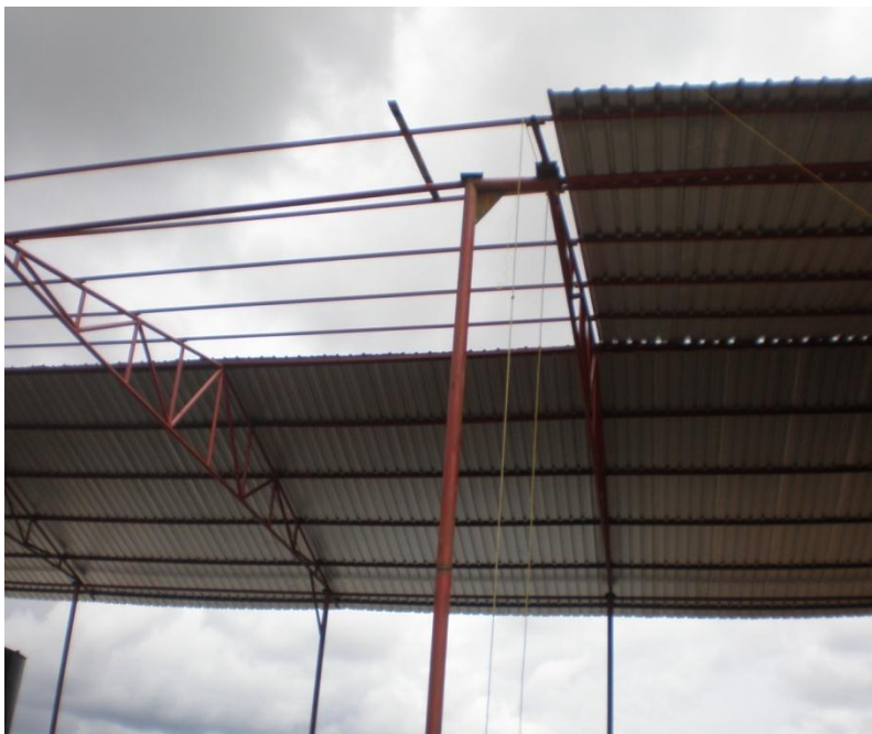
Installation of roofing sheets in progress
