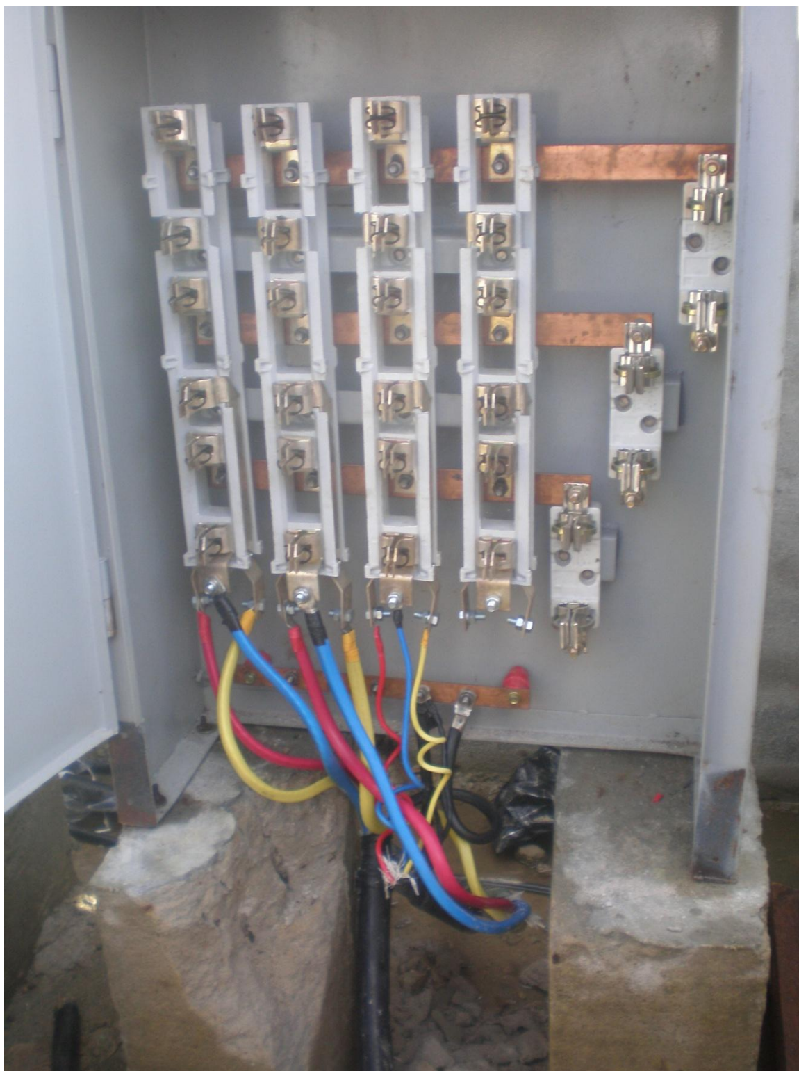
Feeder Pillar installation project for Housing Estate.
